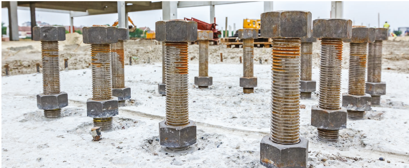
Featured above in the photograph are 'plain finish' hold-down bolts.
